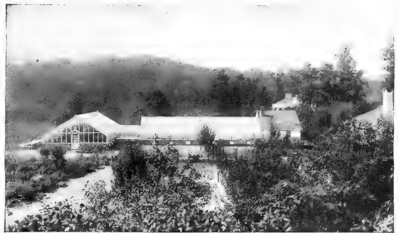
The workroom and adjoining single house were erected for Oliver Iselin, at Glen Head, L. I. Later the large house with its connecting passage was added
